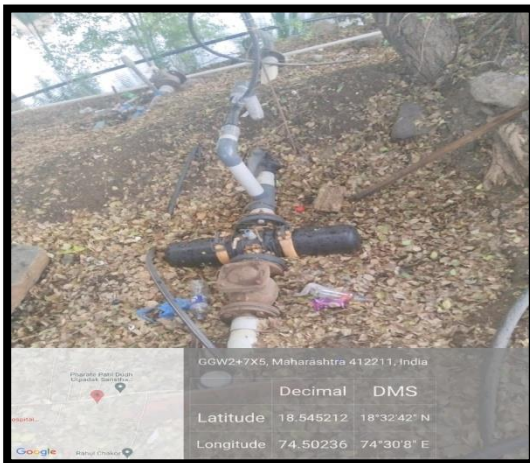
Maintainance of water bodies and distribution system in campus
